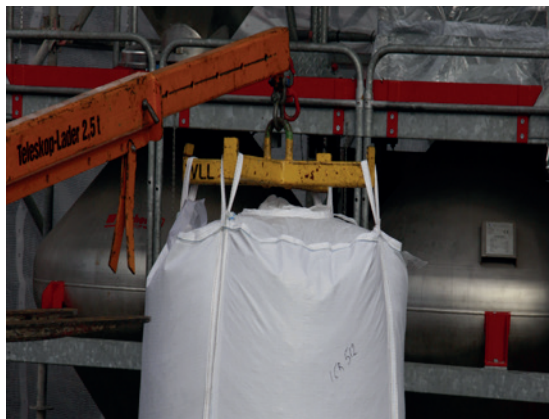
The material is transported from the big bag to the preloading container at the ground level with a forklift truck
